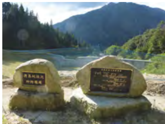
[蛇抜沢砂防堰堤]
